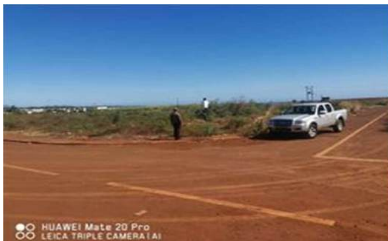
Fig 9. Infrastructure works completed at Cie. De Gros Cailloux Ltee
