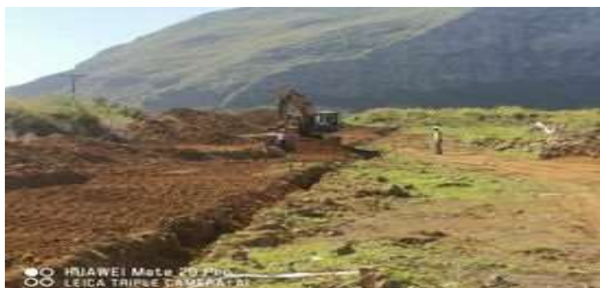
Fig 8. Infrastructure Works in progress at VRS Palma Employees Site – June 2023
